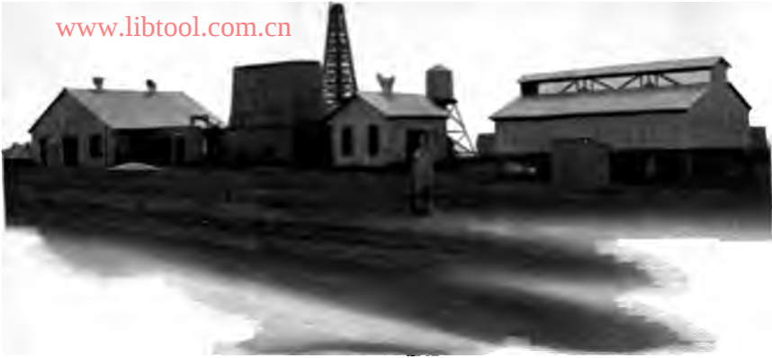
Marland Refining Company Gasoline Plant at Mervine
