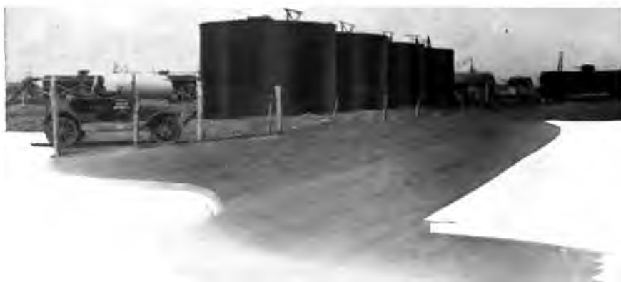
Marland Refining Company loading racks at Covington. Oil is piped to this station from the Garber property, then shipped to the markets in the Company's own tank cars
