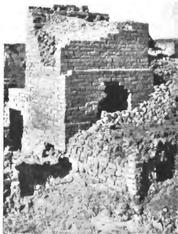
FIG. 71.—Wall of two-ridged bricks in Southern Citadel.
