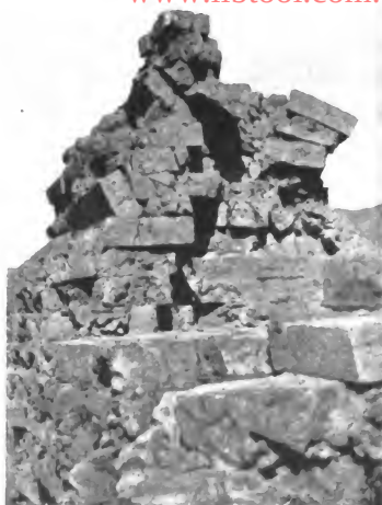
FIG. 61.—Abutments of arches of the Vaulted Building.
