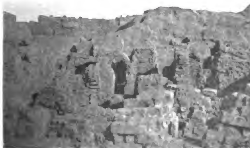
FIG. 60.—Arches of the Vaulted Building.
