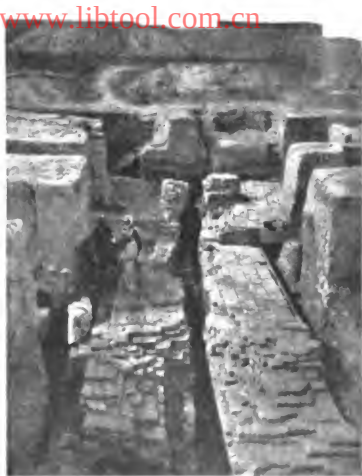
FIG. 97.—Drain through inner city wall.
