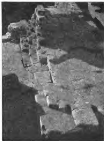
FIG. 22.—Grooved expansion joints at the Ishtar Gate.
