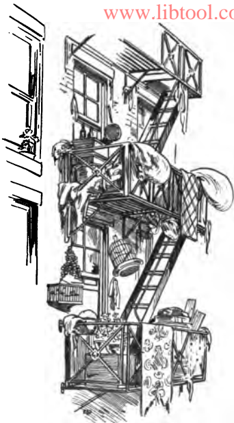
A Blocked-up Fire Escape
