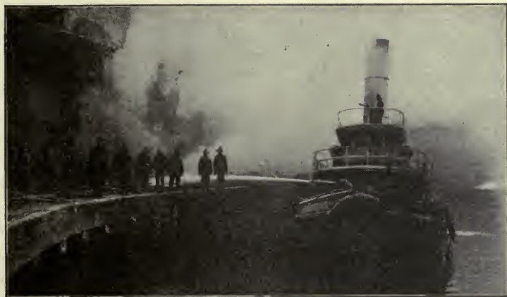
A FIRESHIP SAVING BUILDINGS ON A WHARF
