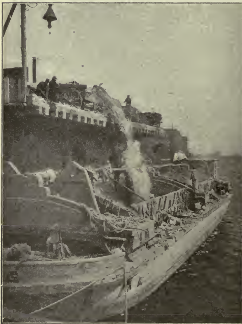
THE DUMPER WHICH RECEIVES THE ASHES
