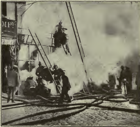
A DIFFICULT FIRE TO SUBDUE
