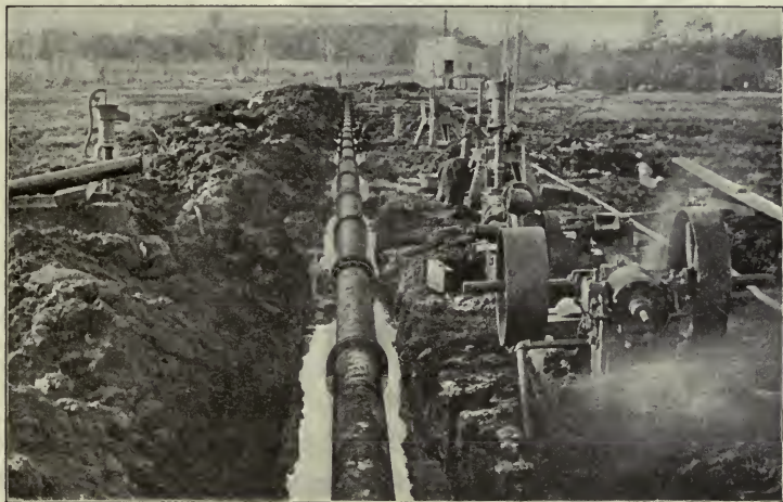
PIPE DRAWING WATER FROM DRIVEN WELLS
