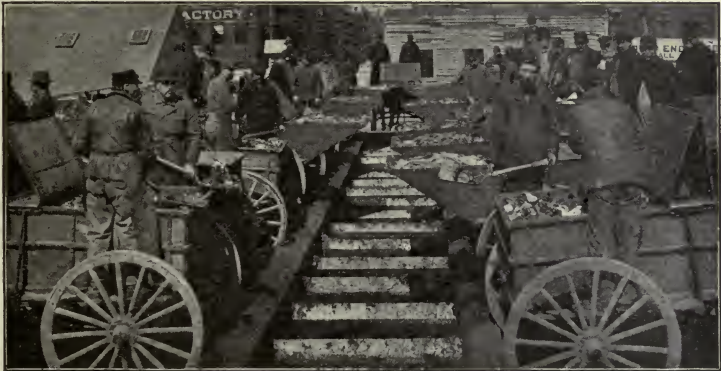
FILLING A DUMPER FROM A BRIDGE
