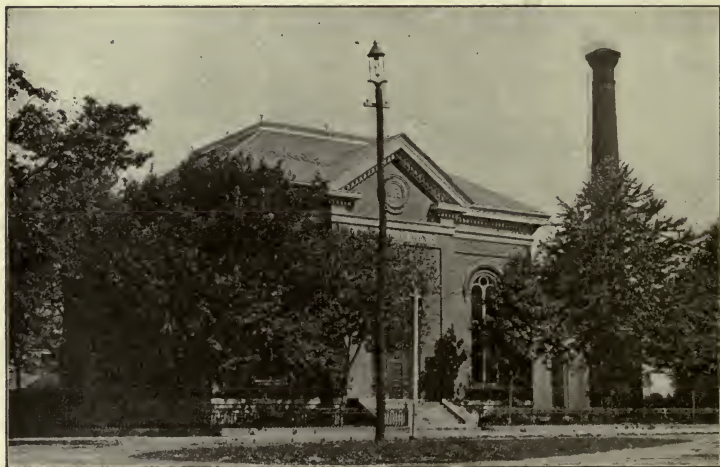
A PUMPING STATION
