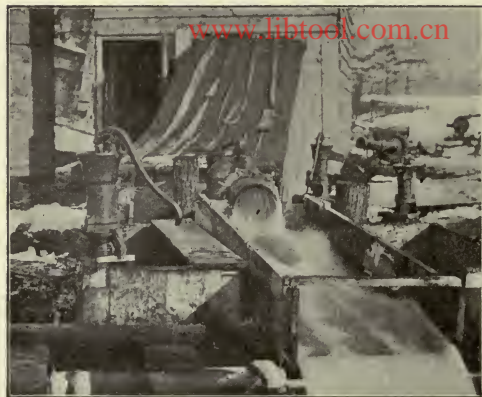
WATER DISCHARGING FROM DRIVEN WELL
