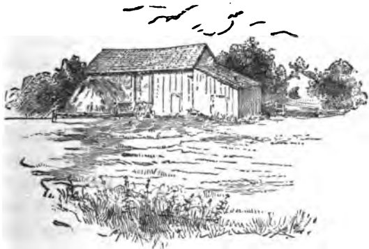
MEADE'S HEADQUARTERS, REAR VIEW.
