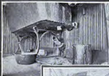
LEAD PIPES OF WASH TUB CUT AWAY ALLOWING SEWER GAS TO ENTER THE APARTMENTS
