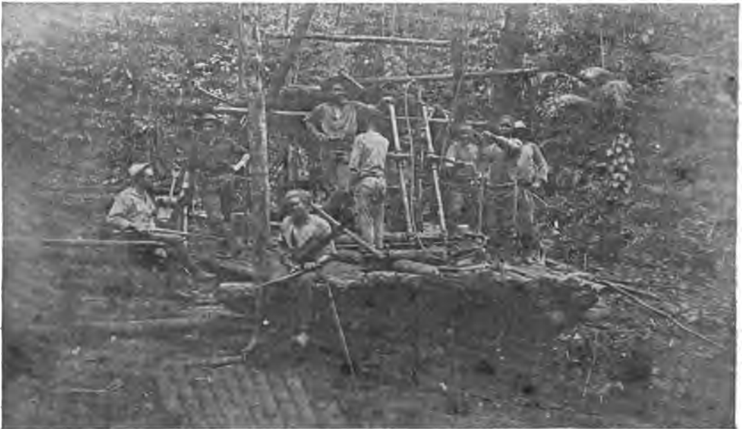
DIAMOND DRILL BORING PARTY.
