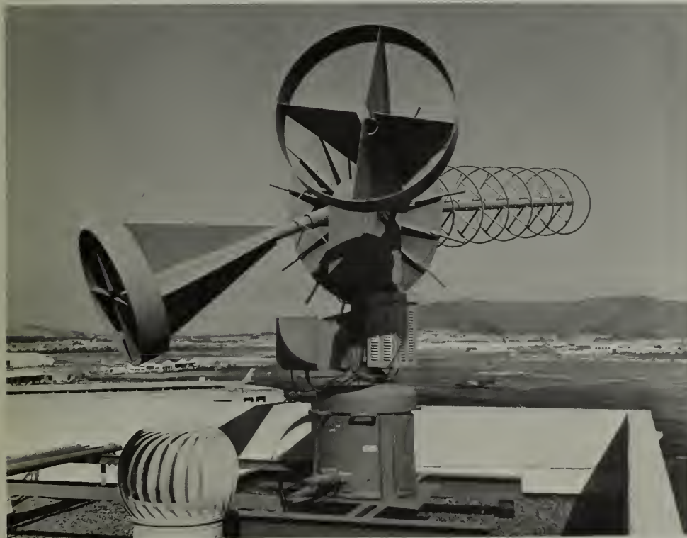
This antennae on the roof of the Central Terminal Building receives weather data from three orbiting satellites. The data is of great assistance to the Weather Bureau in making weather analyses.
