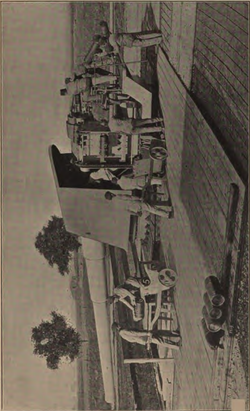
SCHNEIDER-CANET 24 CM. (9.4 IN.) GUN WITH QUICK-LOADING MANUAL ARRANGEMENT.
