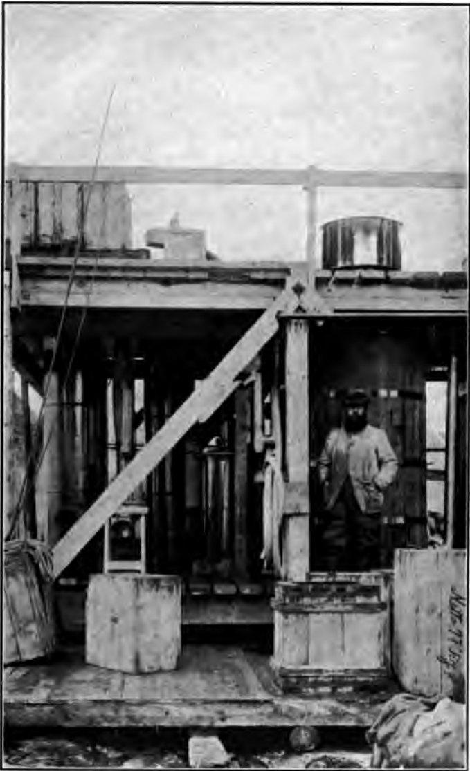
THE HYDROGEN GAS APPARATUS AT CAMP WELLMAN, SPITZBERGEN.
