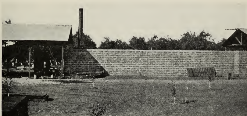
Fig. 1.—One of the first modern air-blast tunnel dehydraters (built in 1921). Note young prune trees in former dry yard.
