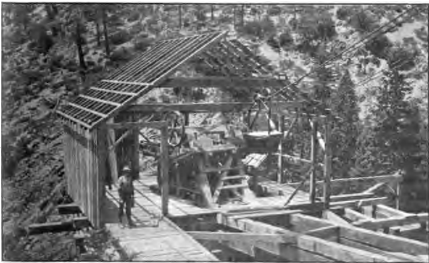
Photo No. 5. Trinity Bonanza King Mine. Automatic tram.
