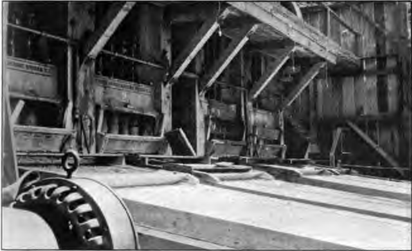
Photo No. 4. Trinity Bonanza King Mine. Interior view, 20-stamp mill.
