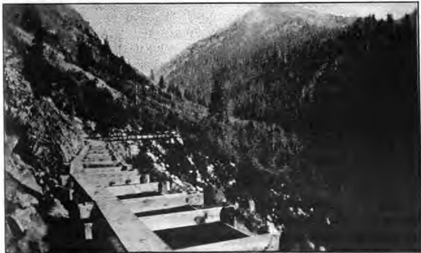
Photo No. 3. Globe Mine; section of flume.
