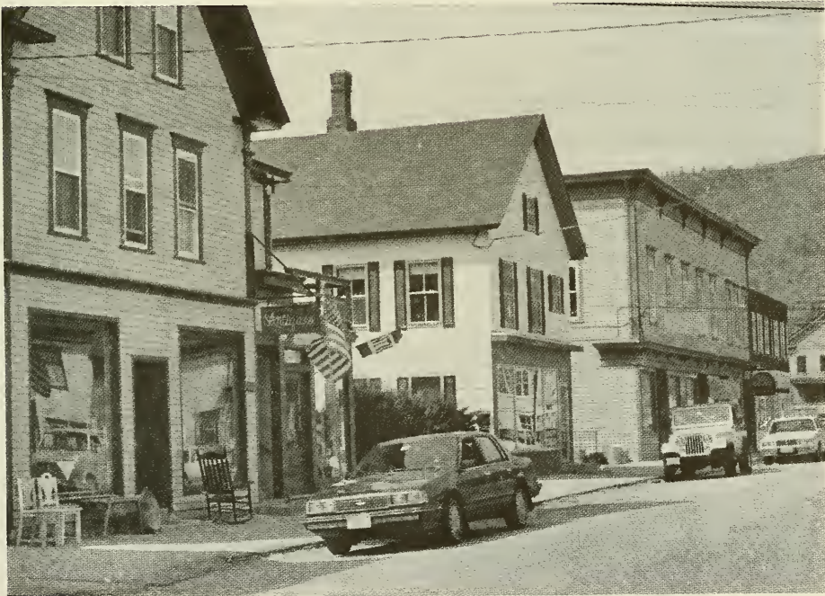
Renovations are slated for Exchange Street in Gorham. LALA DINSMORE photo
