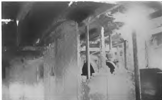
AFTER THE FIRE, LOOKING ACROSS MAIN DECK FROM WOMEN'S STEERAGE.
