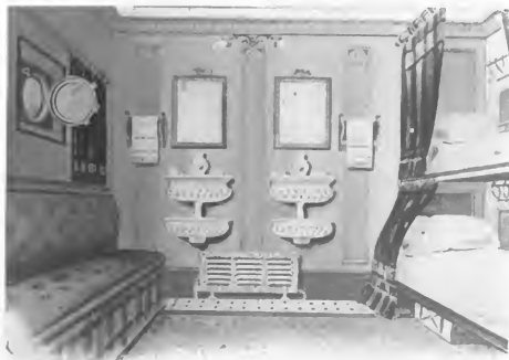
CABIN INTERIOR SHOWING RADIATOR.
