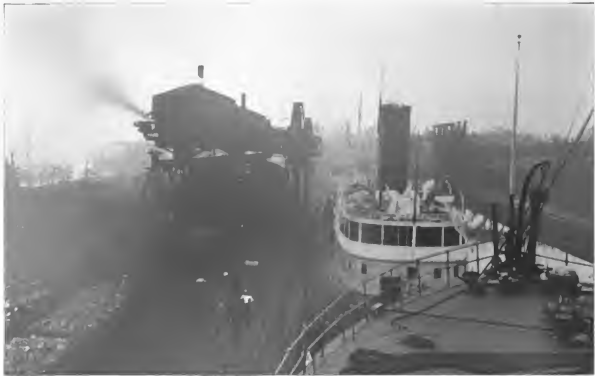
FIG. 2—MINNESOTA DOCK, ASHTABULA HARBOR, O. BROWN SIDE-DUMP UNLOADER, WITH BUCKET TRANSFER SYSTEM.
