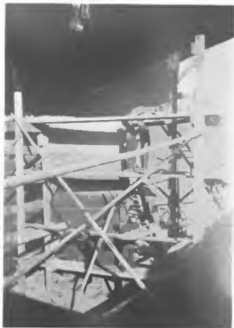
RVETING STERN FRAME IN DRY DOCK.
