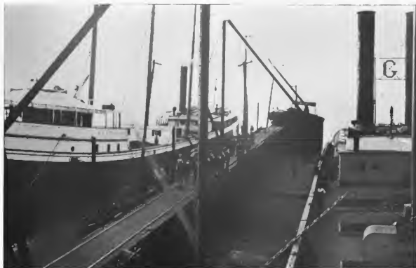
FIG. 1.—B. & O. DOCKS, SANDUSKY, O. CRANE AND BUCKET SYSTEM, THE FIRST TO DISPENSE WITH SHOVELING.
