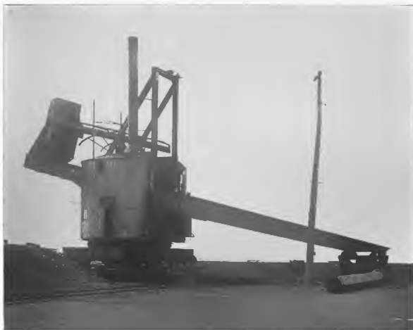
FIG. 3.—M. A. HANNA CO'S DOCKS, ASHUTARULA HARBOR, O. M'MYLER CAR DUMPER, END-DUMP TYPE.
