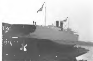
READY FOR LAUNCHING.
