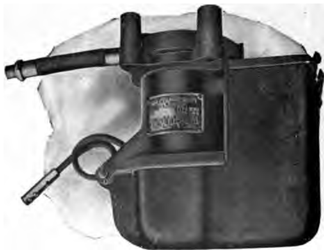
Fig. 476. Air Compressor Governor, Case Closed.
