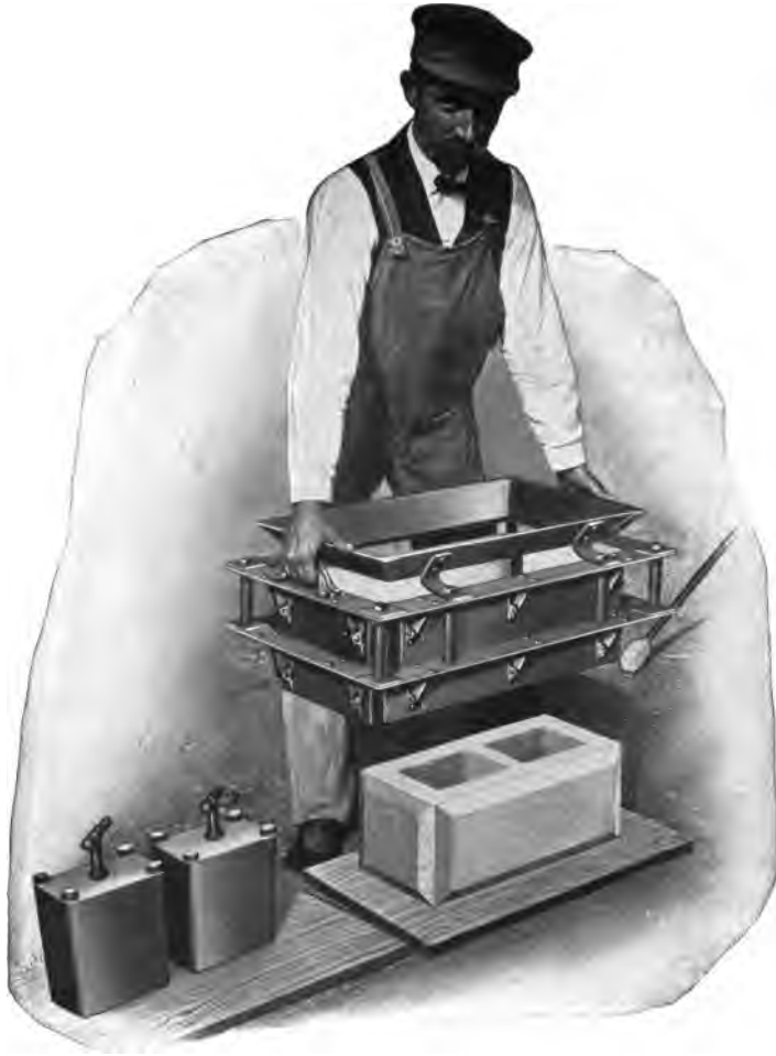
FIG. 16.—Moving the Mold rather than the Block.
