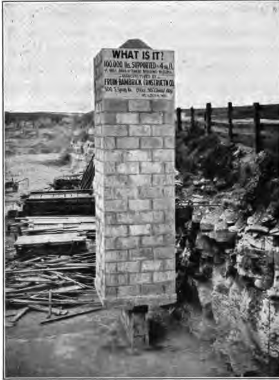
FIG. 24.—Column Demonstrating Compressive and Lateral Strength.
