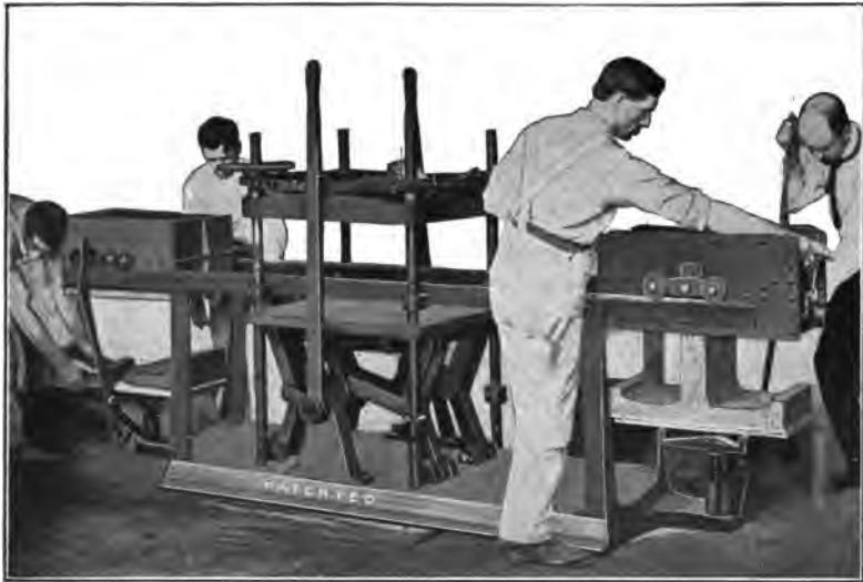
FIG. 19.—Mechanical Press making Two-piece Blocks.
