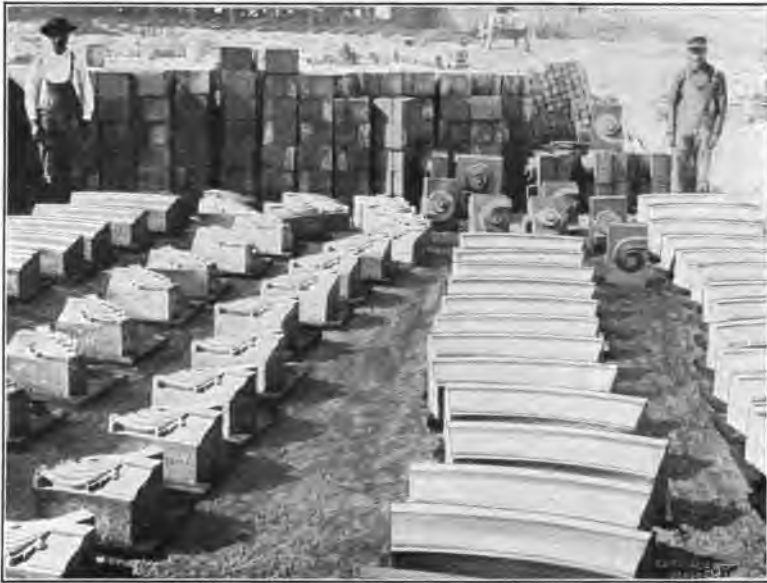
FIG. 12.—Ornamental Work for Chicago Drainage-canal Power-house.
