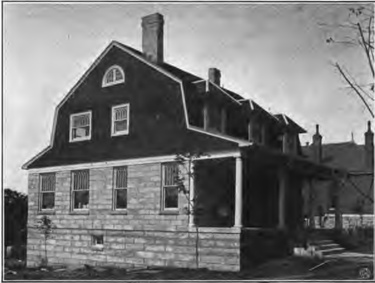
FIG. 29.—Residence, Nashville, Tennessee.
