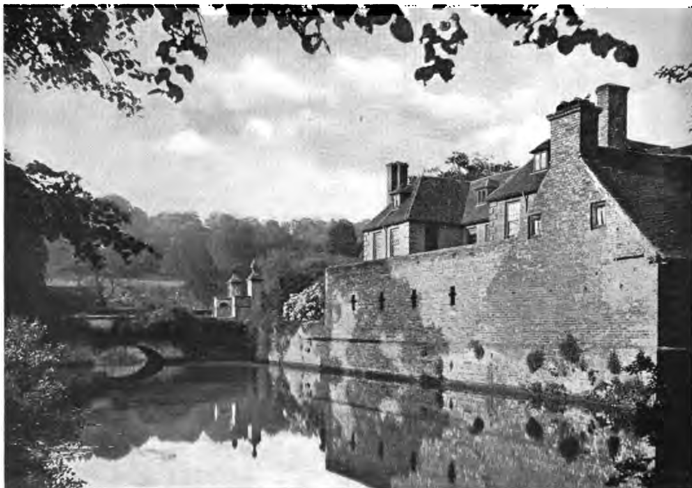
GROOMBRIDGE PLACE, KENT. THE WEST BRIDGE
