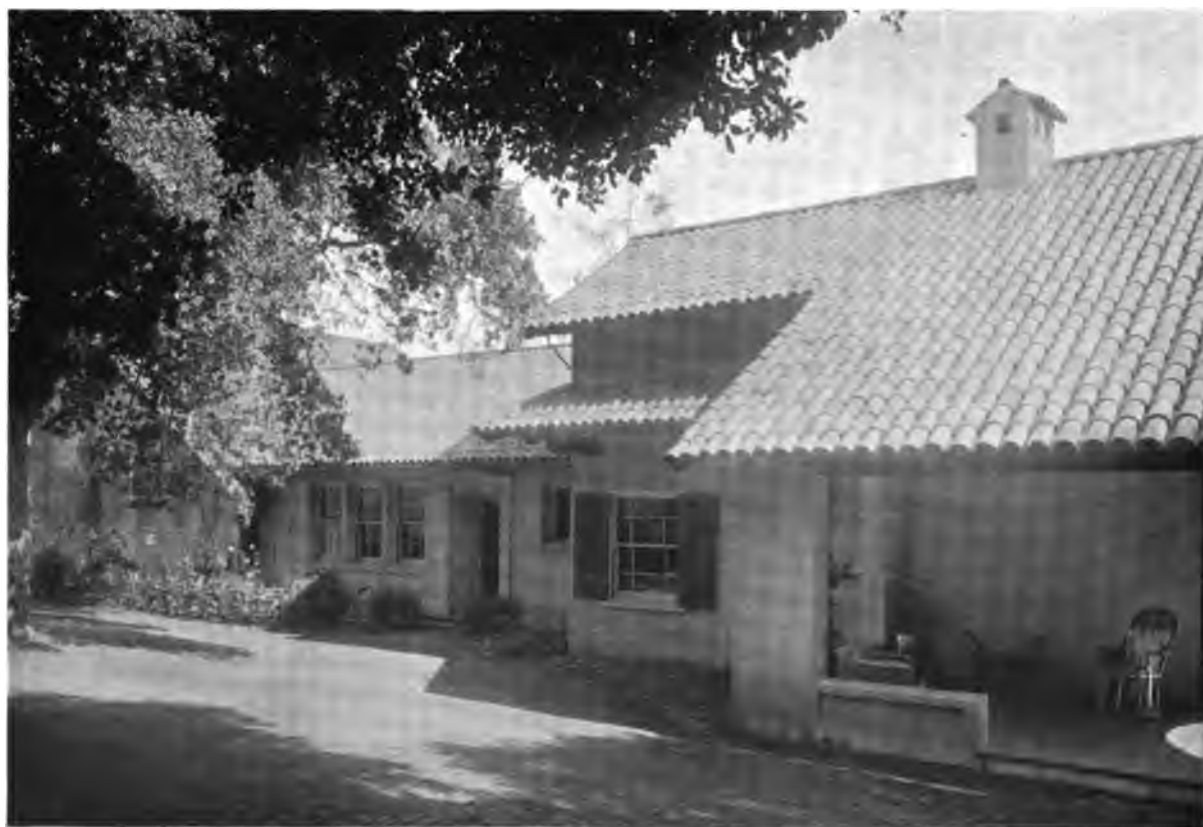
THE REAR OF THE HOUSE
