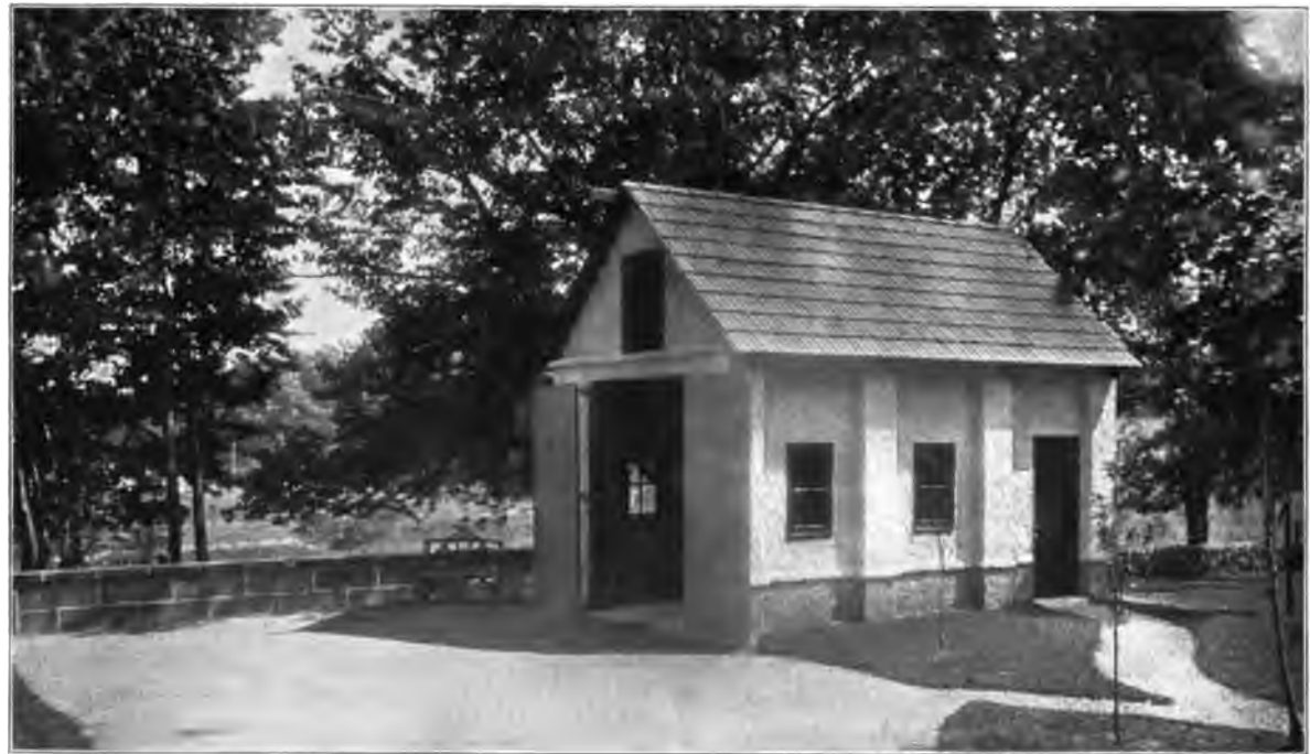
A FIREPROOF GARAGE
