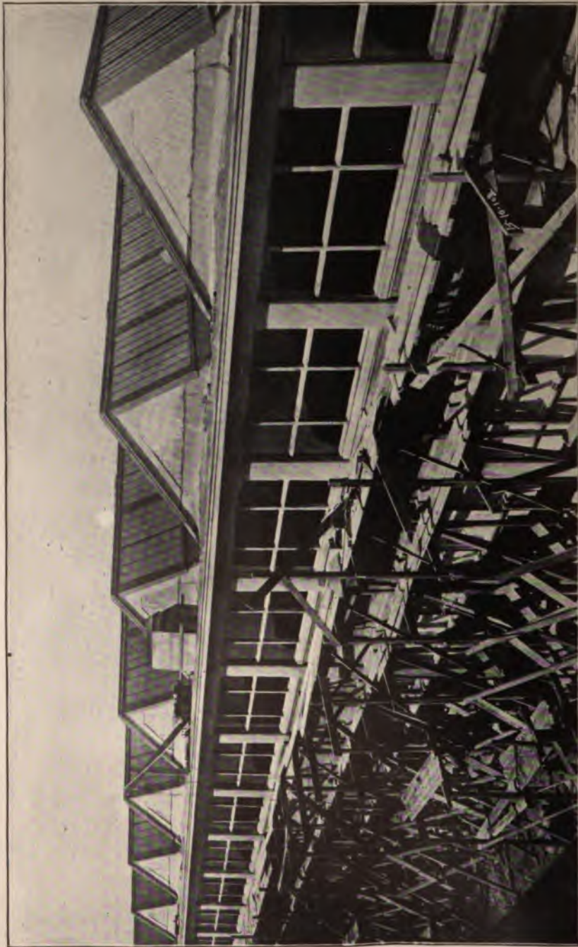
PART OF SAWTOOTH ROOF OF ASSEMBLY BUILDING OF THE GEORGE N. PIERCE COMPANY, BUFFALO, N. Y.
