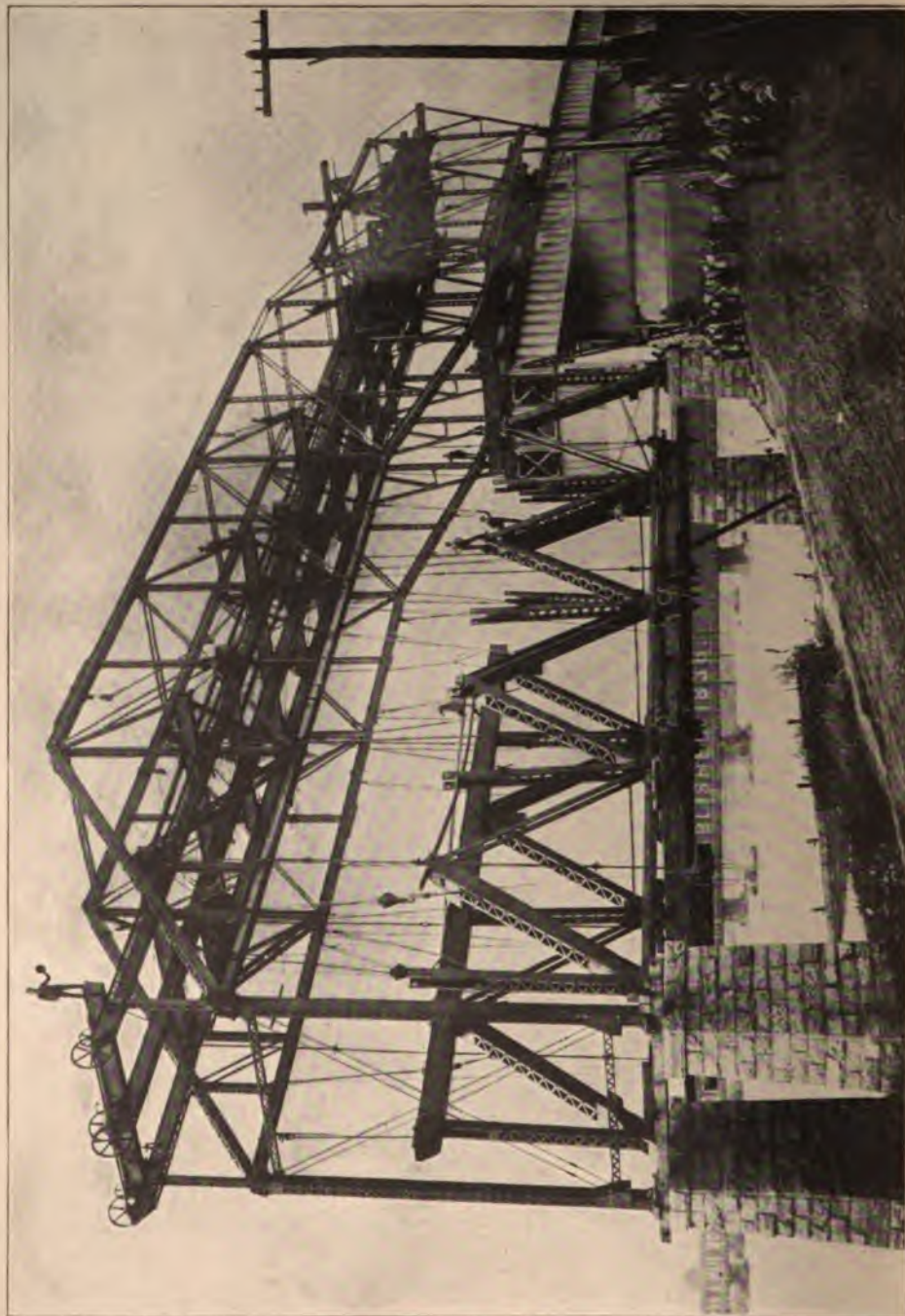
RICHMOND VIADUCT AND TERMINAL RAILWAY AT RICHMOND, VIRGINIA On line of Chesapeake & Ohio Railway. Built in 1900-03. Total length of viaduct 1,859 ft. Property of American Bridge Company.
