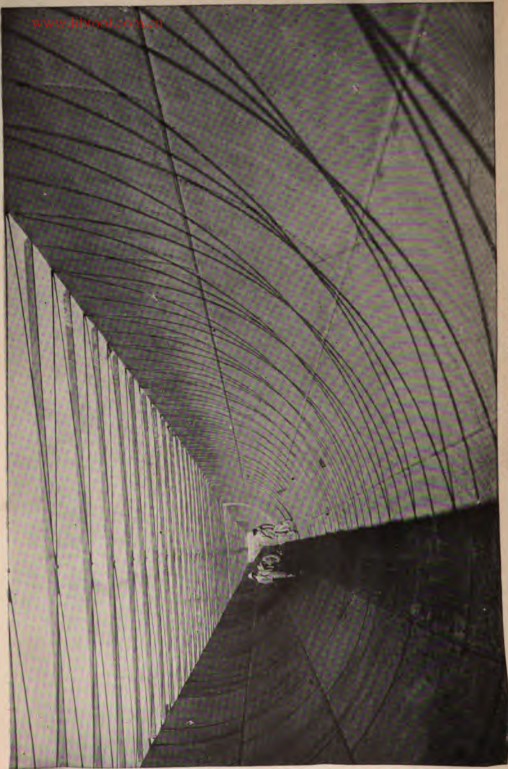
IRRIGATION CANAL BUILT OF STEEL
