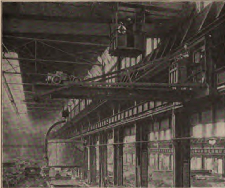
Fig. 100. Wall Jib-Crane, Electrically Operated; Capacity, 10,000 Lbs. Courtesy of Pauling & Harnischfeger, Milwaukee, Wisconsin.
