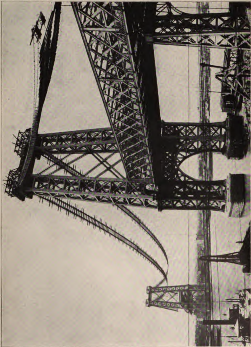
WILLIAMSBURG BRIDGE OVER EAST RIVER BETWEEN MANHATTAN AND BROOKLYN, NEW YORK, UNDER CONSTRUCTION
