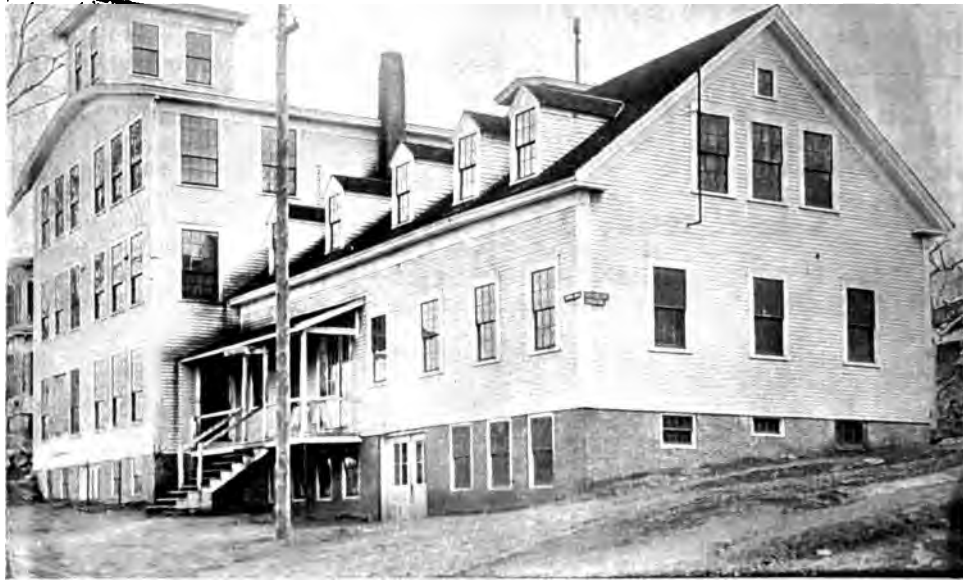
The Huse Machine Shops.
