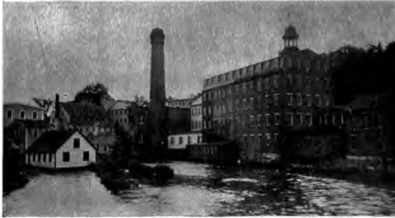
Looking up the River, from Main Street Bridge.
