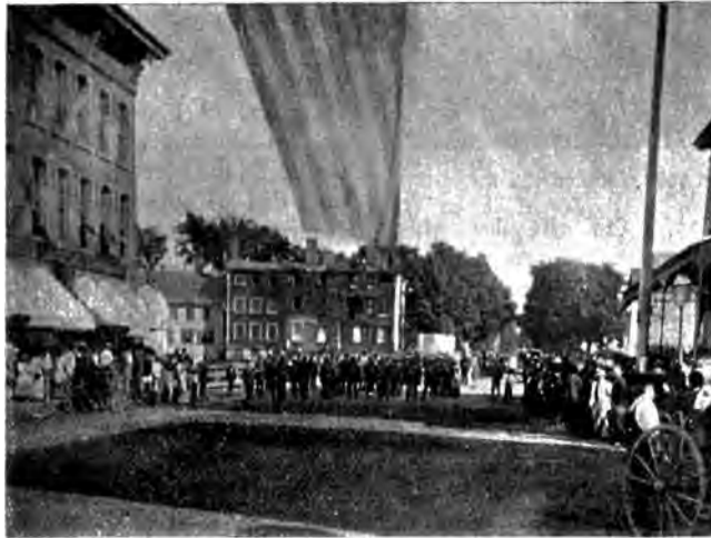
The Old Tremont Building after the First Fire.
