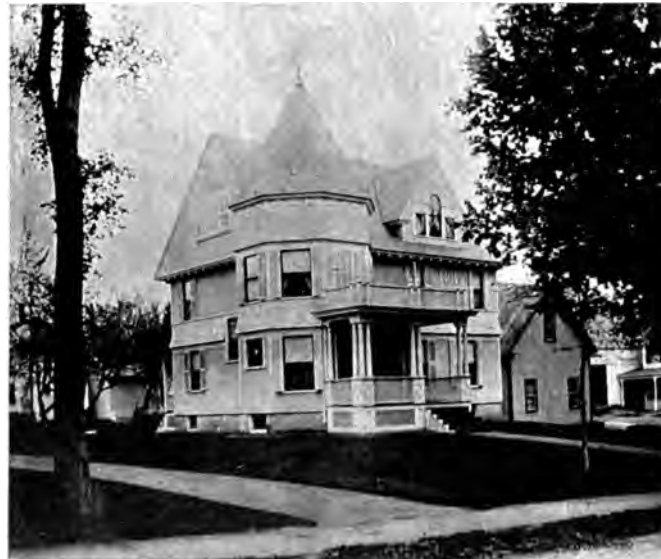
Residence of Harry S. Chase.
