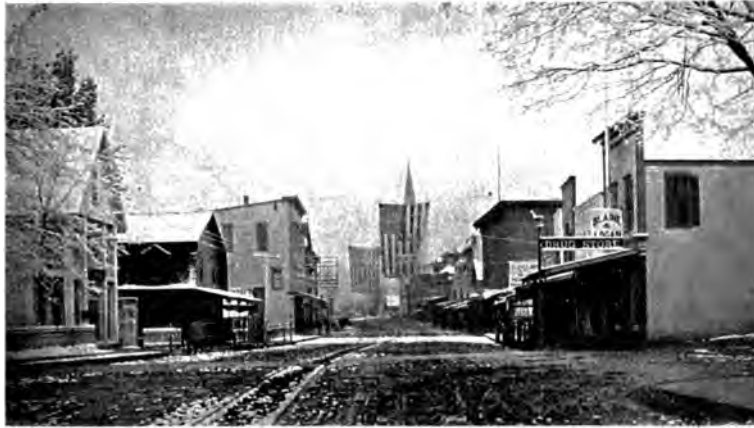
Main Street, before Smith's Brick Block was Erected.
