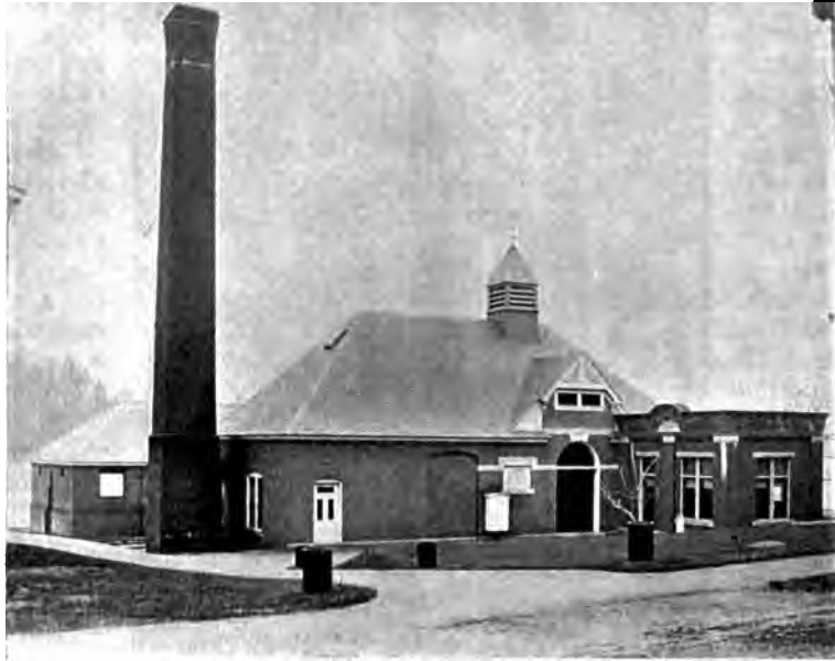
Laconia Pumping Station.
