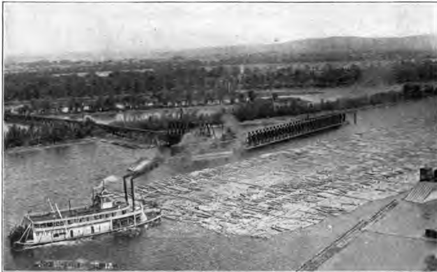
A. LOG RAFT ON THE MISSISSIPPI RIVER AT PRAIRIE DU CHIEN. Note wide-opening of pontoon drawbridge necessary for the passing of large rafts.
