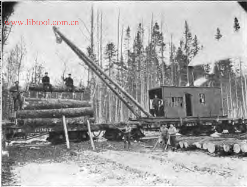
A. STEAM LOG LOADER. CAPACITY 15 CARS PER DAY. Scene near Crandon, Forest Co.
