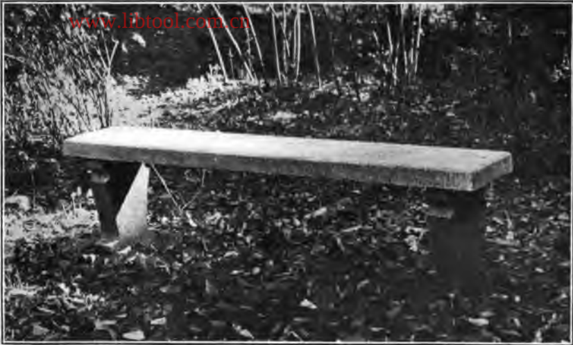
MIDDLESEX FELS RESERVATION. — Concrete Seat.
