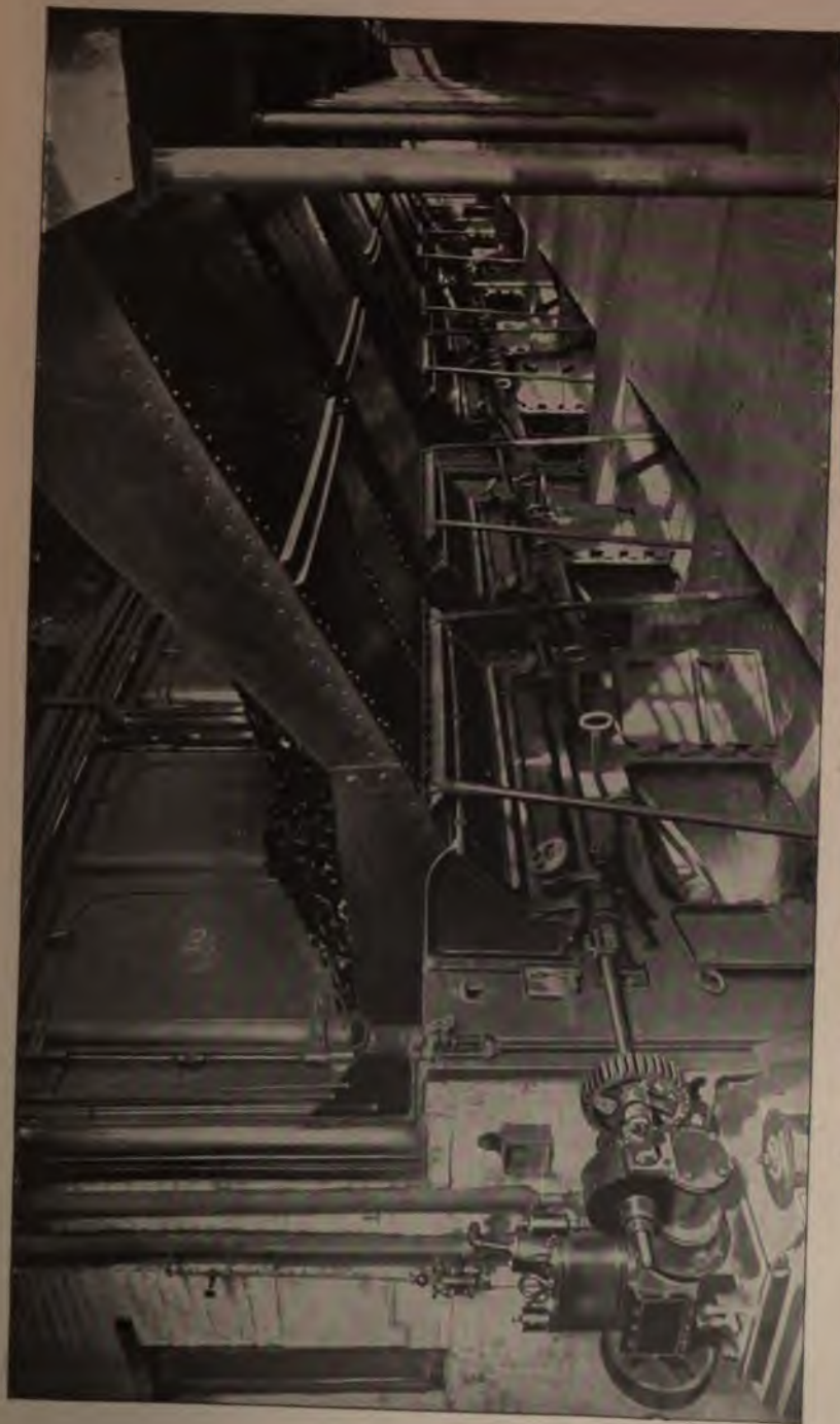
Roney Mechanical Stoker, Showing Coal Delivery Shutes and Operating Engine.
