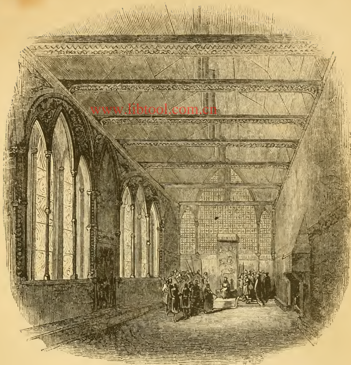
ROOM OF STATE IN THE PALACE.
