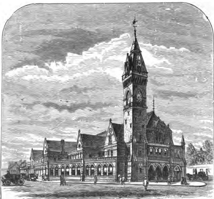
BOSTON AND PROVIDENCE RAILROAD DEPOT, Park Square.
