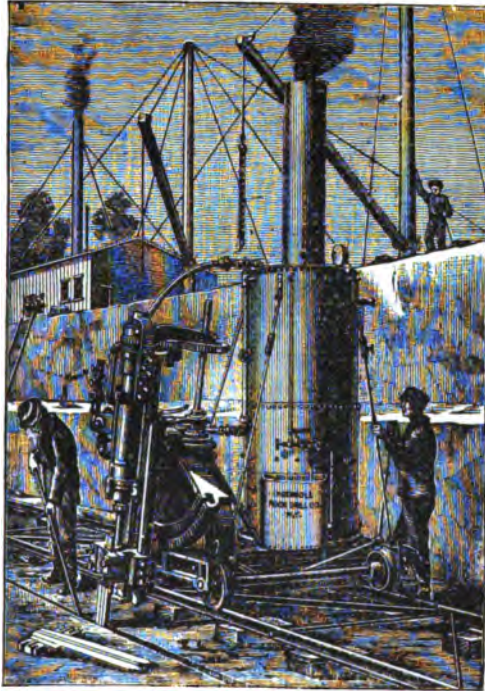
FIG. 12.—SAUNDERS CHANNELLING MACHINE WITH BOILER ATTACHED.
