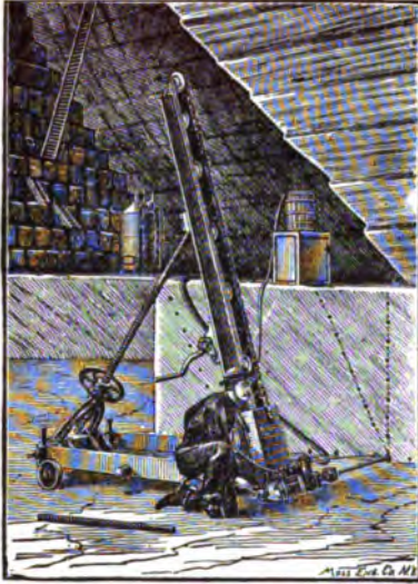
FIG. 17.—INGERSOL STANDARD GADDER AT WORK.
