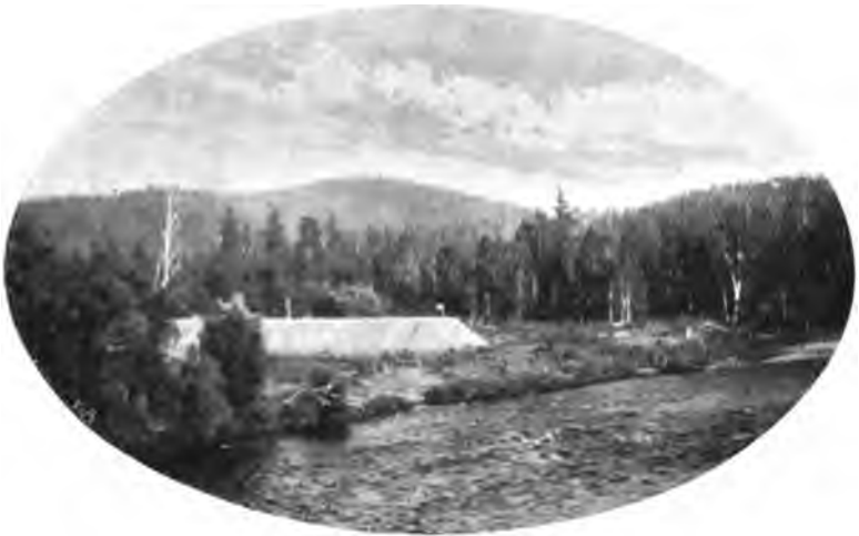
A break in the embankment in Trans-Baikal.
