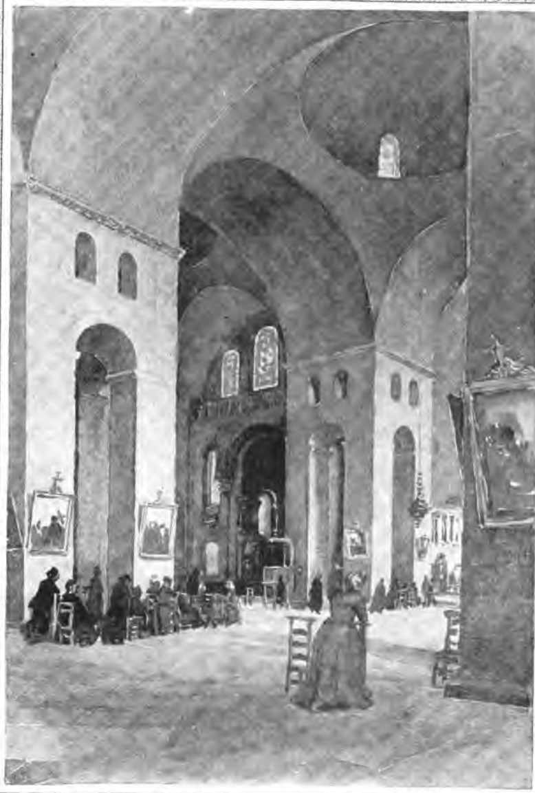
INTERIOR OF THE CATHEDRAL OF ST. FRONT, PÉRIGUEUX
