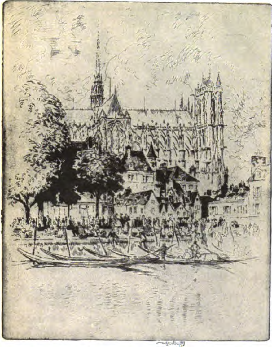
THE CATHEDRAL AS SEEN OVER THE MARKET-PLACE
