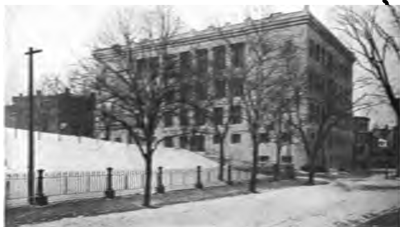
CHARLESTOWN HIGH SCHOOL BOSTON STICKNEY & AUSTIN ARCHITECTS
