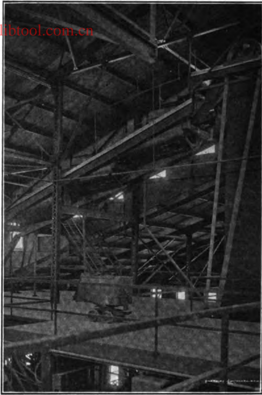
Trommels and Bucket Elevator, Experimental Plant, Colorado School of Mines
