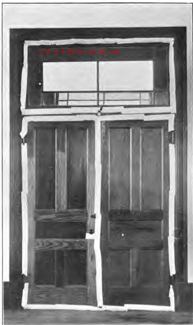
CRACKS AND CREVICES STOPPED WITH PAPER PASTERS.
