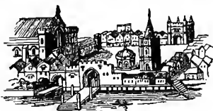
The Palace Yard.
