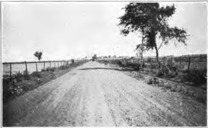
GRAVEL ROAD IN WILSON COUNTY.
