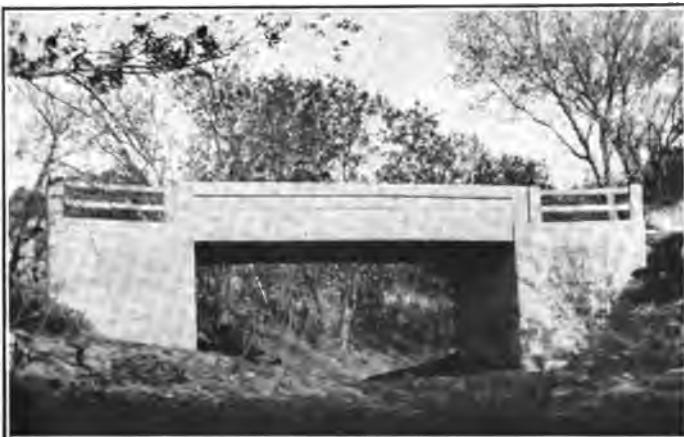
GIRDER BRIDGE WITH RAIL APPROACH.
