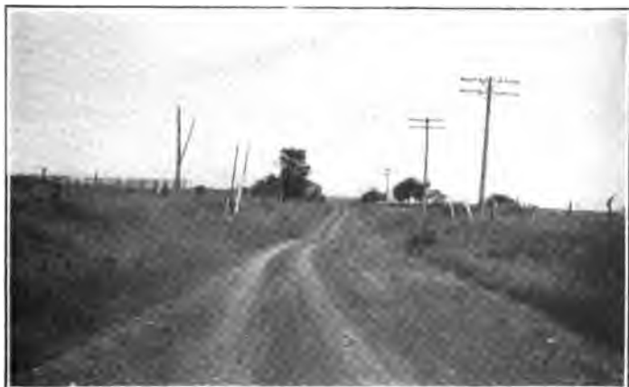
DANGEROUS RAILROAD CROSSINGS.
