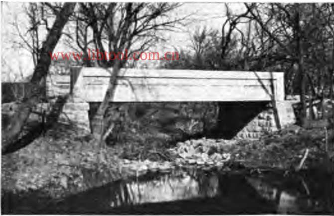
A FINE SPECIMEN OF A THROUGH-GIRDER BRIDGE.
