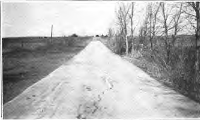
CONCRETE OVERFLOW ROAD IN HARPER COUNTY.
