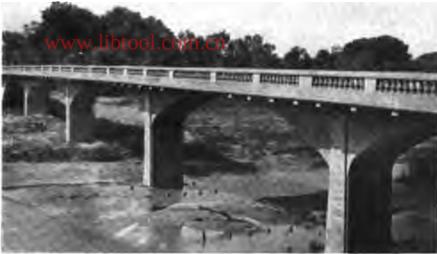
HANOVER BRIDGE, WASHINGTON COUNTY.
