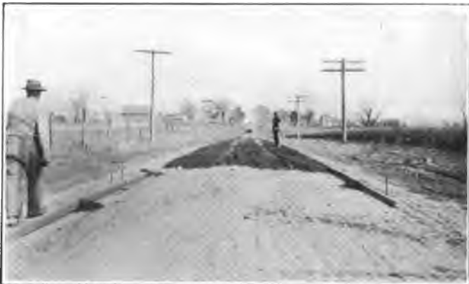
LAYING A GRAVEL ROAD IN ANDERSON COUNTY.
