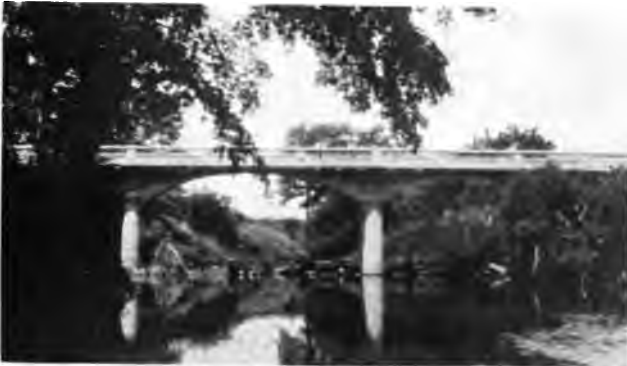
OSWEGO BRIDGE, LABETTE COUNTY.
