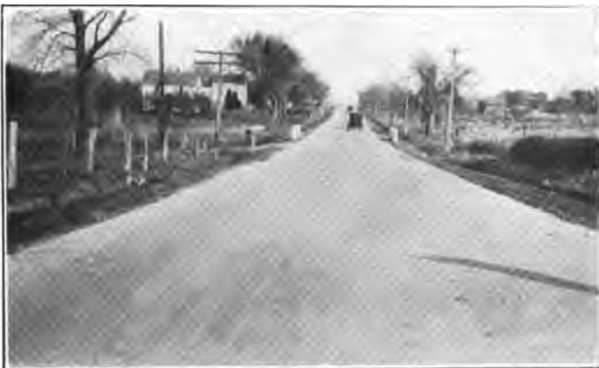
WATERBOUND MACADAM IN SHAWNEE COUNTY.
