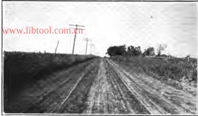
A GRADED AND DRAGGED EARTH ROAD IN WILSON COUNTY.
