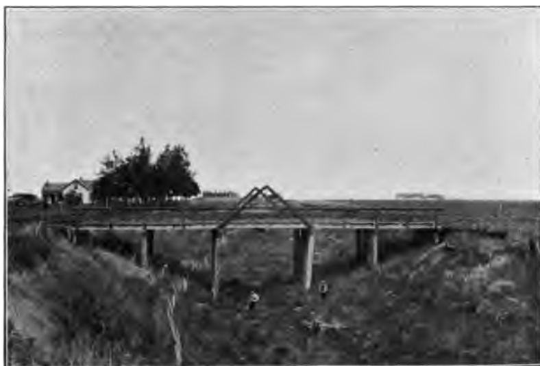
Road Ditch Eroded in Four Years. Ditch Discharging Into Red River of the North. Township 140, Range 48.
