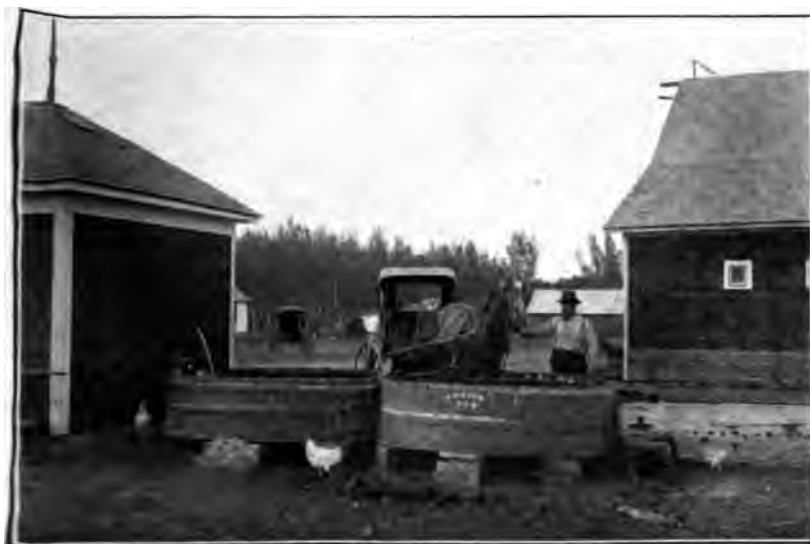
Flowing Well and Tanks, Red River Valley.
