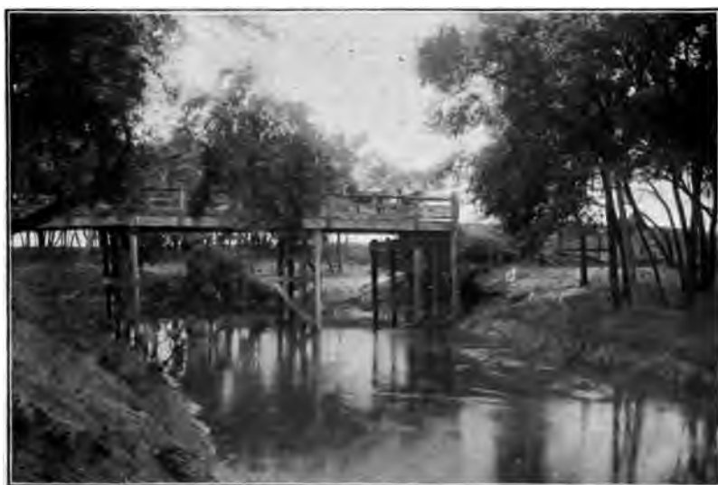
Bridge Over Sheyenne River at Haggart Station.
