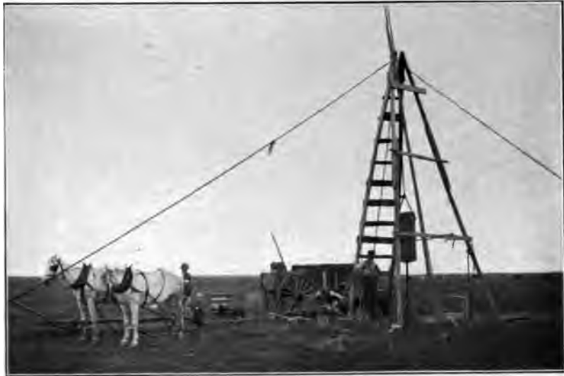
Digging Well—Driving Pipe.
