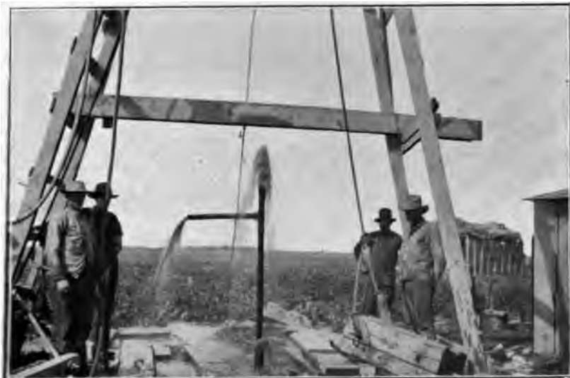
Flowing Well. Just Struck, Trott Farm, Casselton Quadrangle. (Depth 418 feet. Flow at first, 4,000 bbls. per day. Section 10, Township 140, Range 53.)
