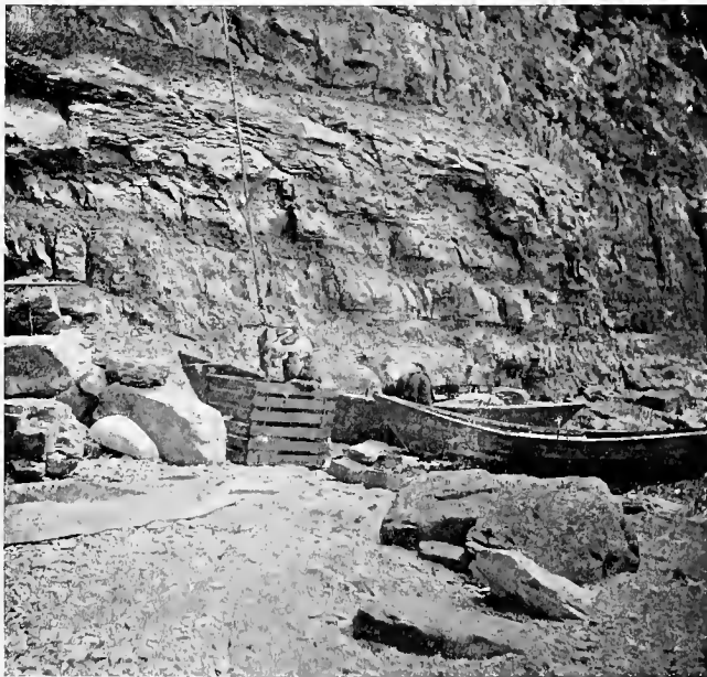
83. The landing at the base of the Rock, showing crate.
