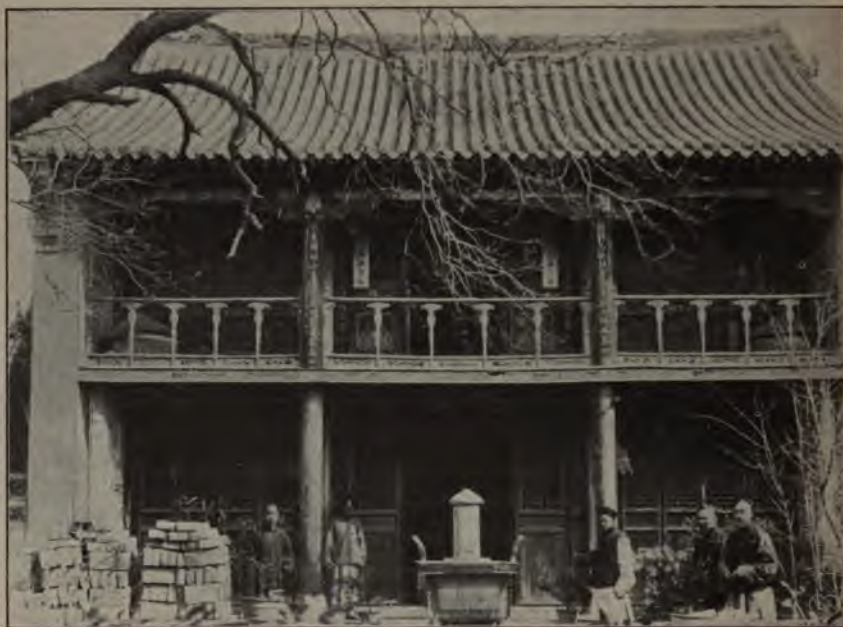
Tempel Simati in Jentschoufu.
