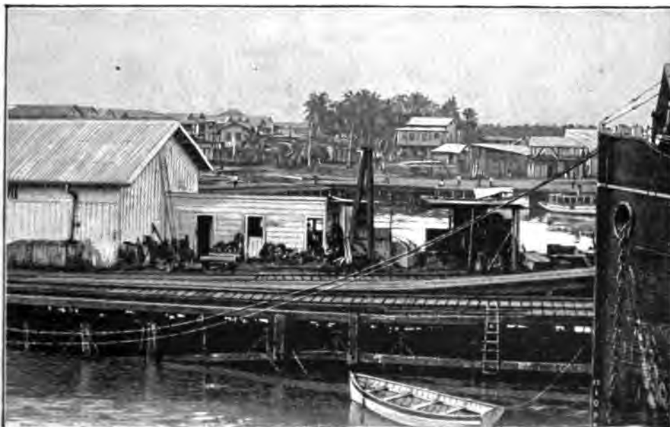
WHARF AT COLON.
