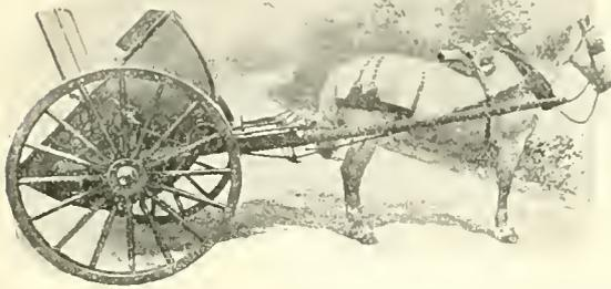
FIG. 3943.—Garbage Cart at an Angle for Washing or Easy Loading.
