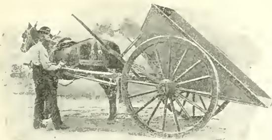
FIG. 3944.—"Columbian" Dumping Cart showing Use of Dumping Lever.
