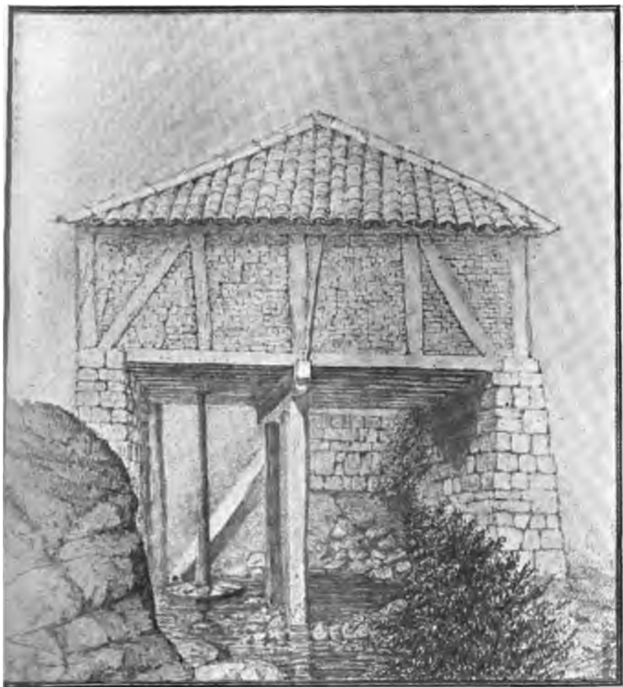
WATER-MILL WITH HORIZONTAL WHEEL.
