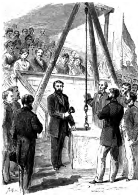
LAYING CORNER STONE OF CHURCH—GENEVA.
