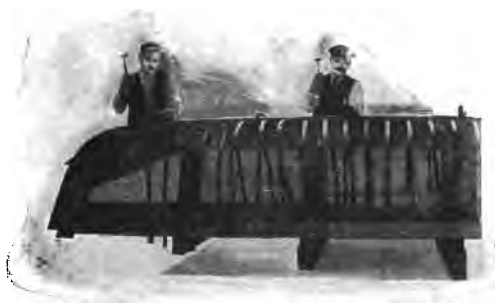
Placing Steel Hull Over Frame.
