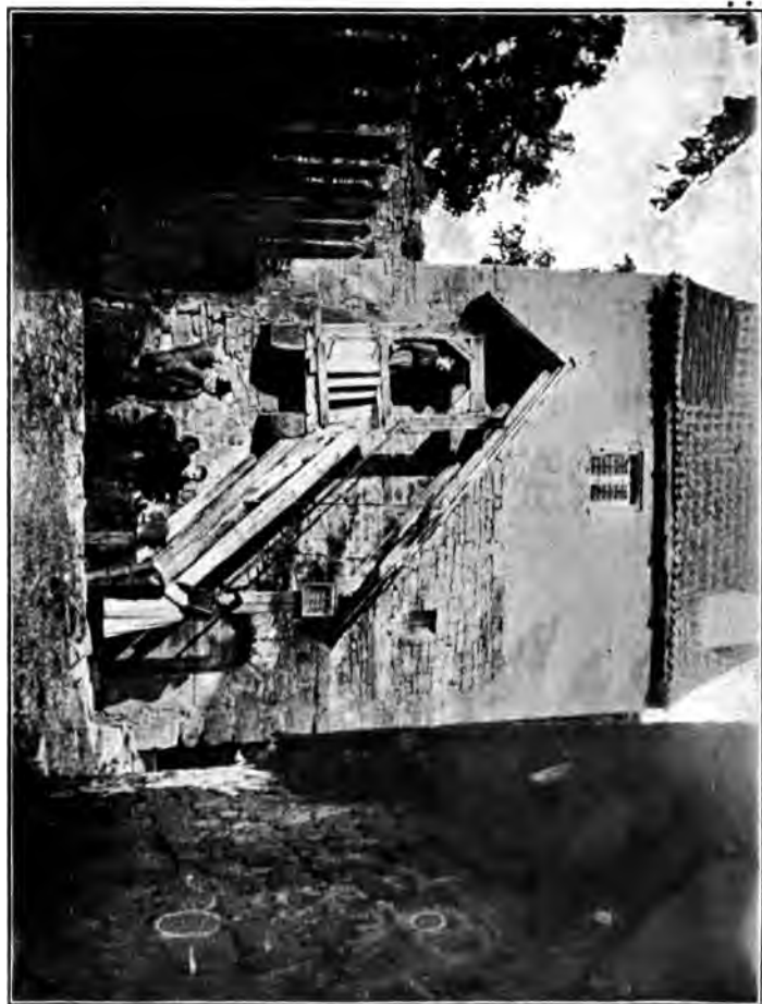
ENTRANCE TO WALL TOWER IN SOMMERHAUSEN (1903).
