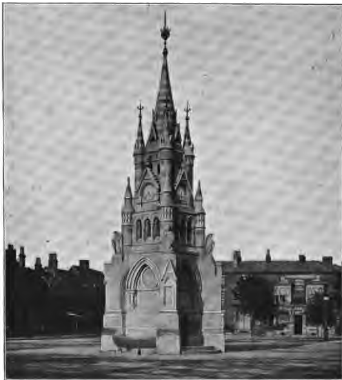
THE AMERICAN FOUNTAIN AND CLOCK-TOWER, STRATFORD.
