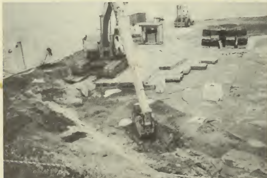
Inside the enclosure, radioactive waste is dug out of the holding basin and placed into cubic yard boxes for shipment to a licensed LLRW disposal site in Utah. (Photo courtesy Starmet Corp.)
