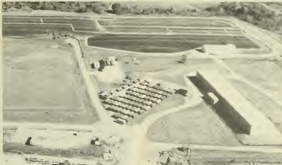
A view of the LLRW disposal area showing the trench covers, including plastic membranes, used at West Valley to minimize water intrusion into LLRW disposal trenches.
