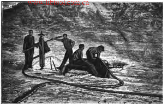
Drilling for blast in a Kansas mine.
