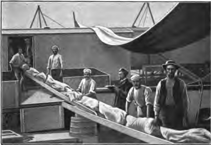
Slide into the cold storage chamber of a steamer.
