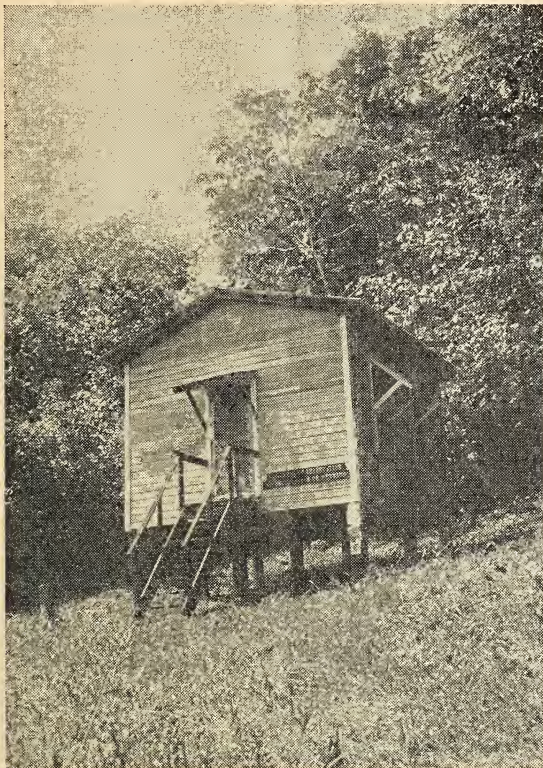
FIGURE 4.—Rest house on Barro Colorado Island, Canal Zone, constructed in 1926 of timbers impregnated with either coal-tar cresote or zinc chloride.
