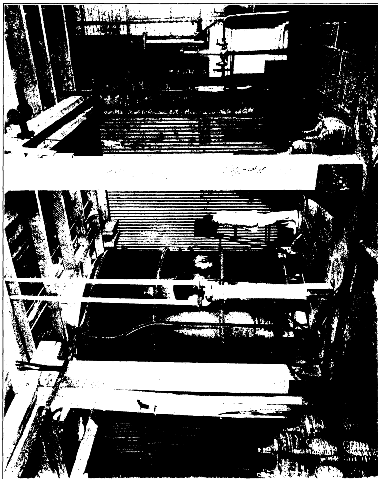
PLATE VII. A RECTIFYING STILL IN YNCHAUSTI AND COMPANY'S PLANT.
