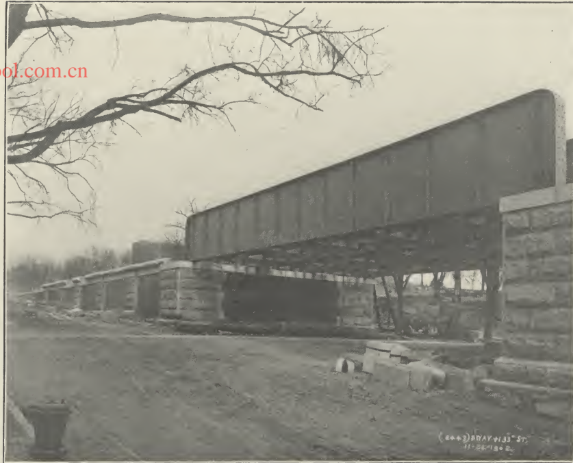
MANHATTAN VALLEY VIADUCT APPROACH.
