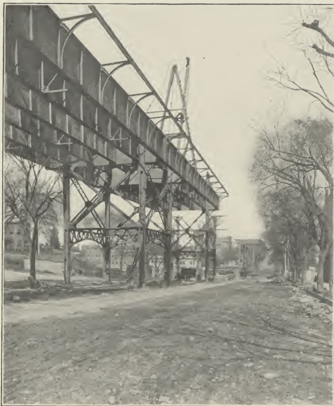
MANHATTAN VALLEY VIADUCT.
