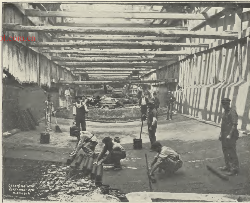
WATERPROOFING INVERT, 149TH STREET.
