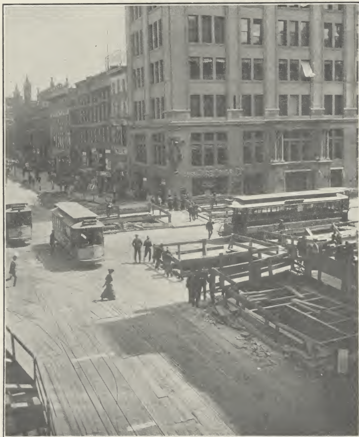
INTERSECTION OF FOURTH AVENUE AND 23D STREET.
