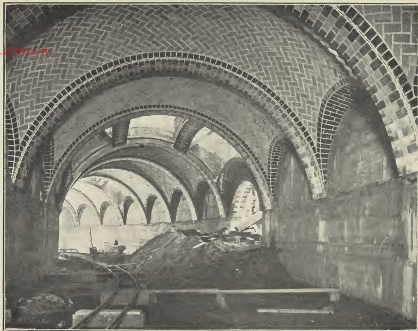
CITY HALL STATION.
