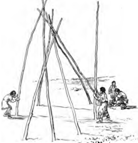
Building an Indian tent
