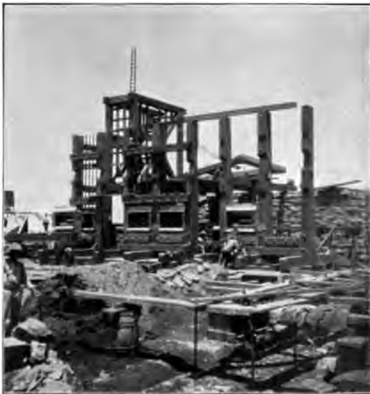
ERECTING A STAMP MILL ON THE RAND, SOUTH AFRICA.
