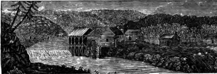
FIRST MILL IN OHIO.*
